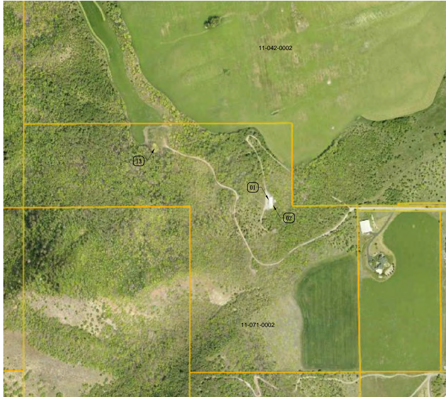
2 AERIAL SITE PHOTO SCALE: NA G101
